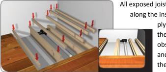
All exposed joists will now need a noggin or batten running along the inside of the joist to accommodate the new
