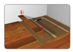
If you are left with a gap between the edge of the shower tray and the start of the original flooring, this should be filled with a piece of the flooring that you removed in Step 4 and securely screwed down onto the new plywood.
